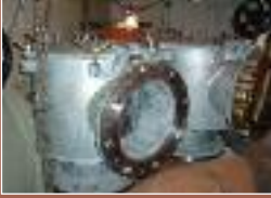
DN 350 bilge water filter Sea-water filters for engine cooling
